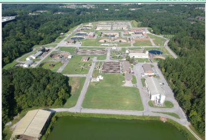
The Cahaba River WRF is a 12 MGD plant located in south Jefferson County that primarily serves the Hoover area. It is an activated sludge plant with a 5-stage biological nutrient removal (BNR) system. The WRF also has the ability to receive flow and/or send flow through the Al Seier pump station to the Valley Creek WRF.
